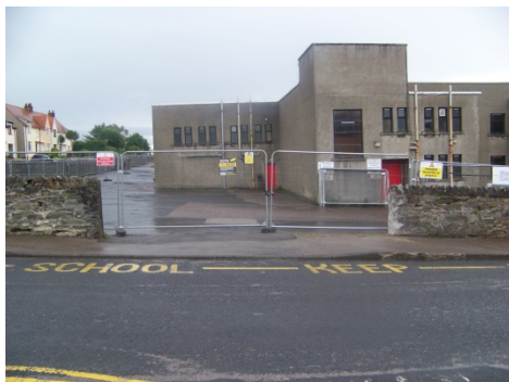
6a Existing school buildings to be demolished
