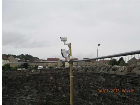
9 Site security CCTV cameras
