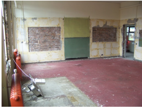
5a Pre- Demolition - "soft strip" of existing buildings
