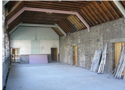
4 Existing 1881 school building "retained shell"
