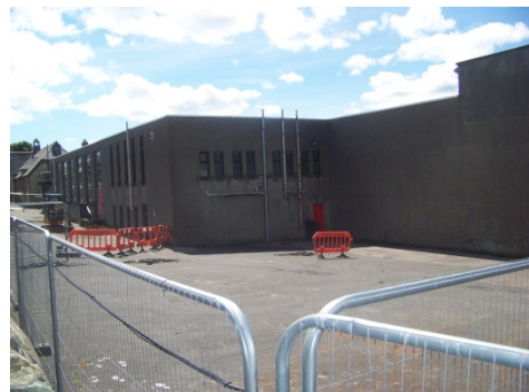
6b Existing school buildings to be demolished
